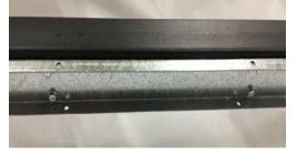
Mount offset bracket to the frame using 4 #8X1/2" hex head screws. <u>If these are on the lower bar it is important to mount these before the frames are set.</u> Bracket should be centered on the pair of power openings.
