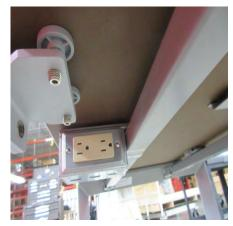
L-111-LS box mounts to A-117 bracket at required a justable location on bracket using 3 10-32X3/16 THMS.
